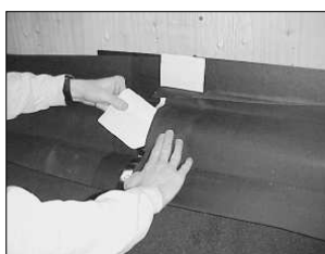
Step 7. Fold over the end lap, carefully peel away to release paper, smooth the end lap into position on the seam tape.
