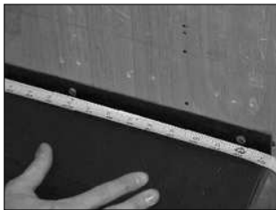
Step 4. Fold over cover membrane to expose concealed nailing strip, squeeze bellows to proper position, nail concealed nailing strip to top of other curb or to chalk line on wall, nailing 4" oc on the curb or 8" oc on the wall.
