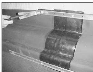
Step 10. Fasten the termination bar, included, along the top and/or bottom of the cover membrane.
