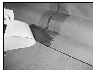
Step 8. Prime each end, place the splice tab equally over the full width of each end of the cover membrane.
