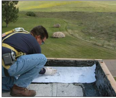
2. Embed PermaFlash Scream
