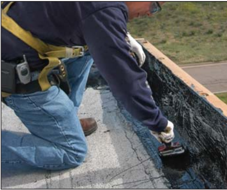
4. Coat entire scrim area
