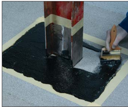
2. Apply base coat
