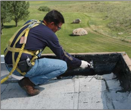
1. Apply base coat
