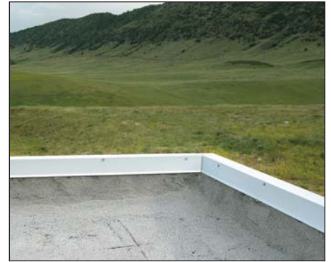
6. Finished wall flashing
