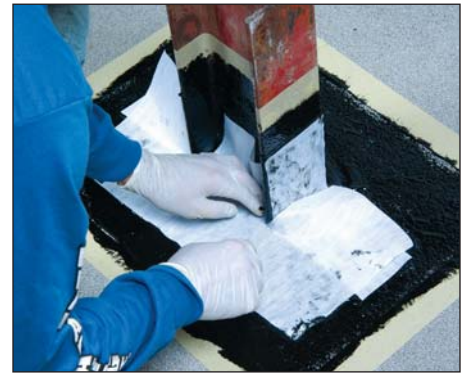
3. Embed PermaFlash Scream
