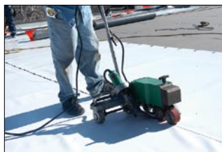
Hot-air weld field seams.
