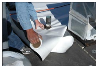
Custom flash penetrations, then treat with a hot-air welder.
