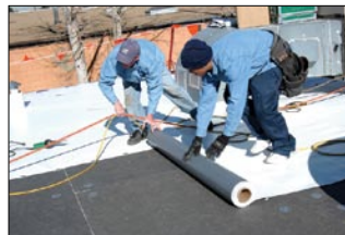
Roll JM PVC or JM TPO single ply membrane into place.
