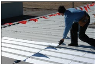
Install insulation between ribs with JM ENRGY 3® polyisocyanurate.
