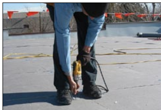
Lay approved cover board (i.e., Invinsa Roof Board) over the insulation and ribs, then mechanically fasten.
